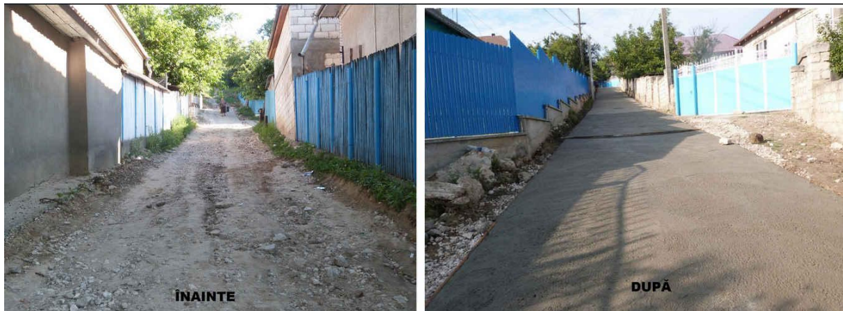
Costești, before and after
