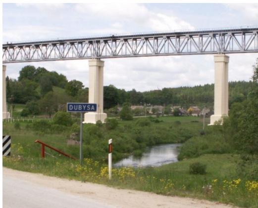
Lyduvenai Bridge above the Dubysa
