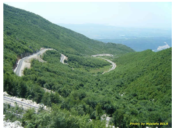
High-angle shot of the road to Mali i Krujës
